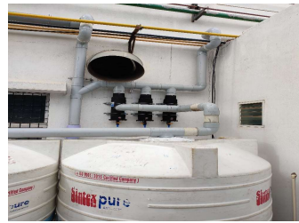
Rainwater harvesting system in INDO-MIM
