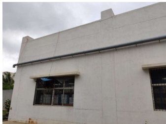
Rainwater harvesting system in INDO-MIM
