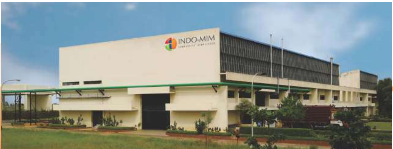
Doddaballapur Manufacturing & Finishing Facility, Bangalore
